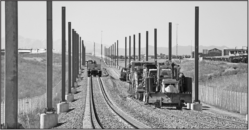
The RTD line to the Denver airport under construction on the east side of Pena Boulevard in Denver on October 6, 2013. – Photo © 2013 Dave Schaaf.
