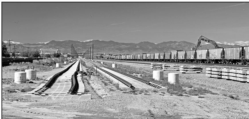
The RTD line to the Denver airport under construction on the west side of Havana Street in Denver on October 6, 2013. One new track is for the UP and two are for RTD. – Photo © 2013 Dave Schaaf.
